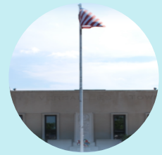
North Versailles Township Building
